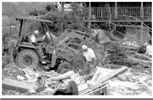
Holston Disaster Response Team works clearing storm debris.
