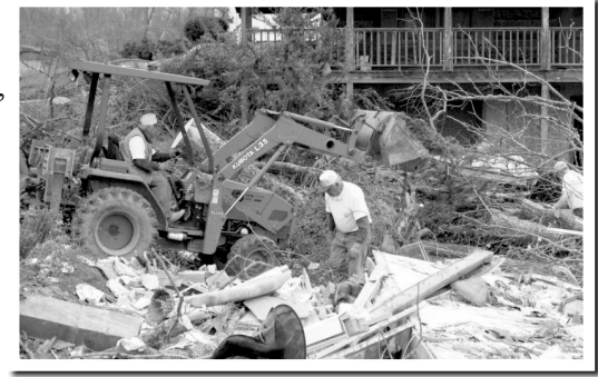
Holston Disaster Response Team works clearing storm debris.
